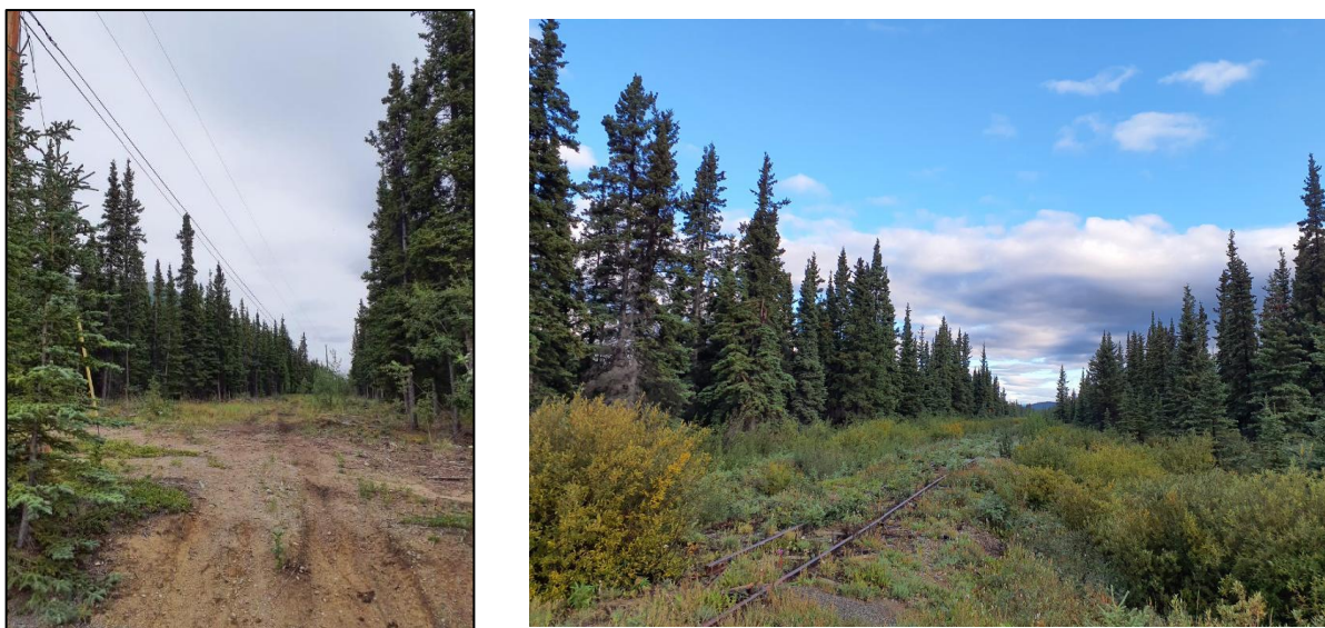
Figure 10: Examples of good right-of-way vegetation management on ATCO corridors in the Choutla subdivision, and along a decommissioned portion of the railway right of way north of the Watson subdivision.
