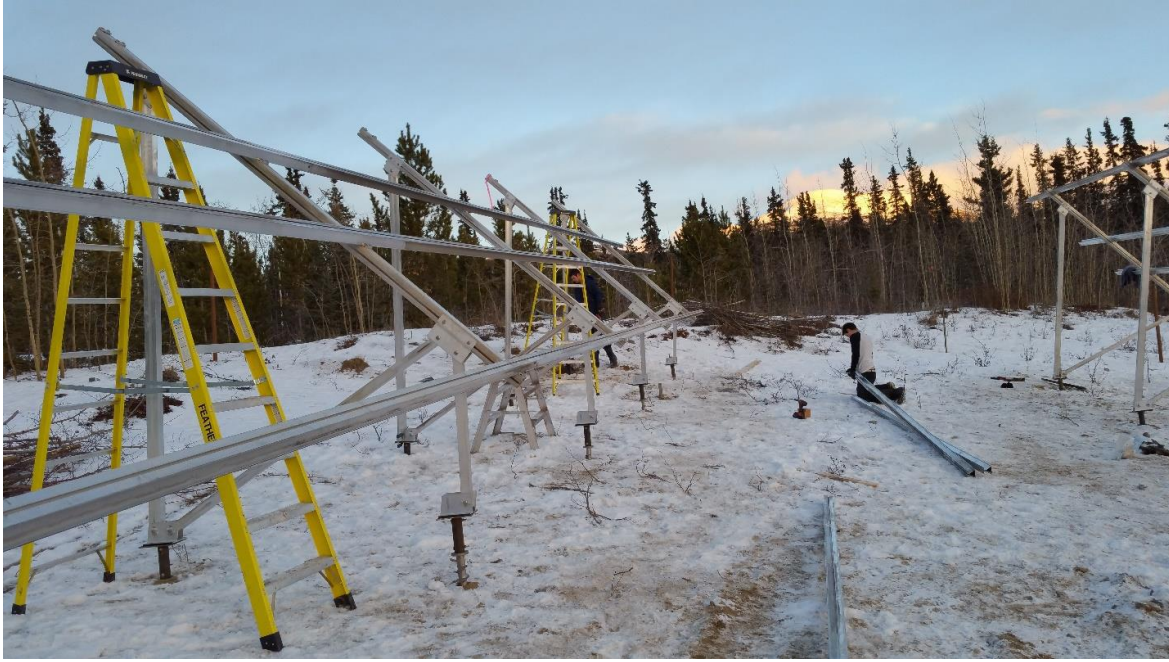
Figure 10 : Array foundation installation and levelling [photo credit: Total North Communications]
