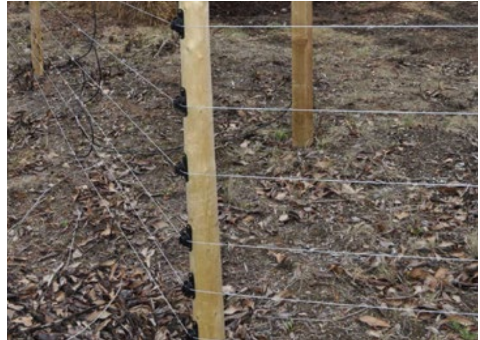
Post and insulators
