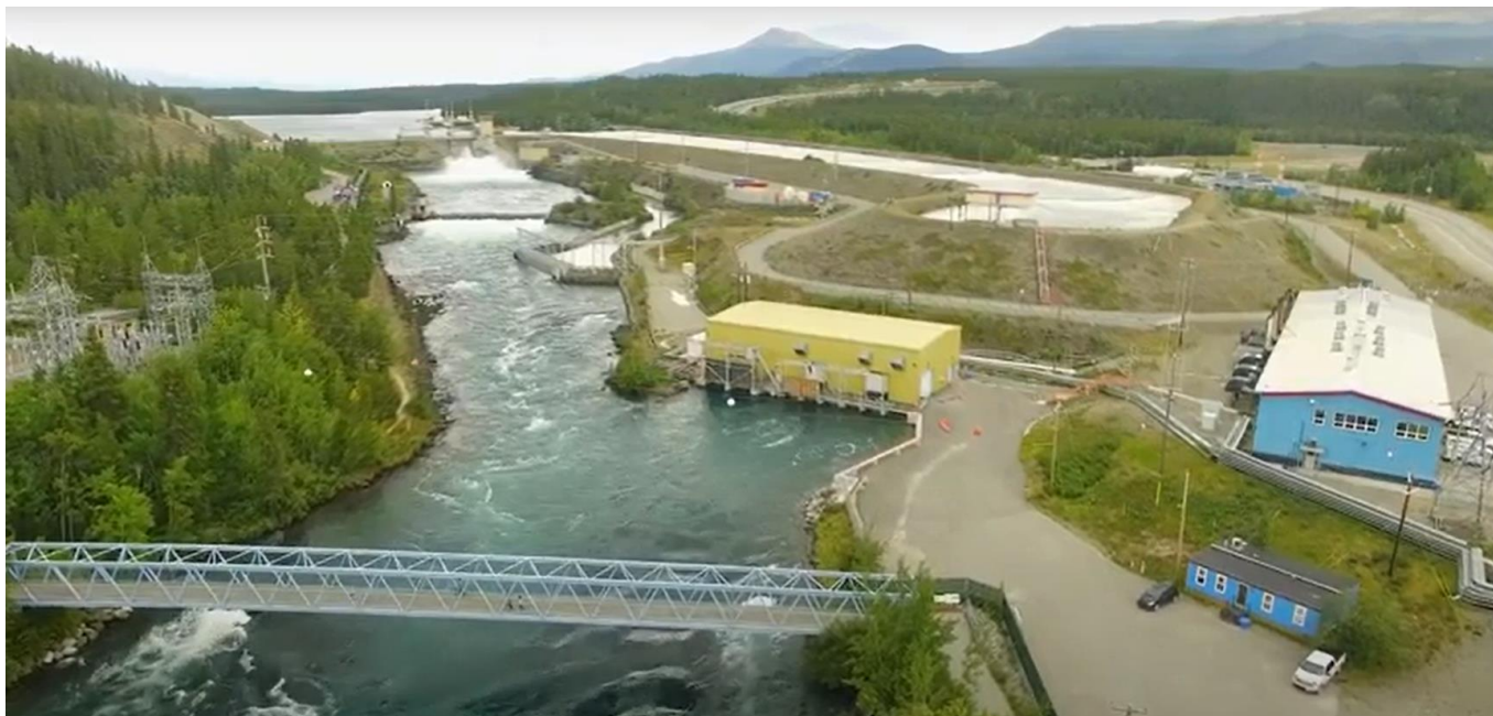
Figure 2. Current Yukon major hydroelectric project example: Whitehorse Hydro Plant (Yukon Energy).
