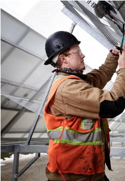
Solvest employee installing solar panels.
