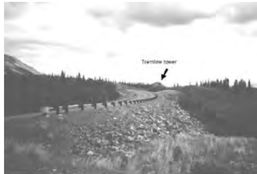
Figure 10: View of tramline tower from proposed pull-off.
