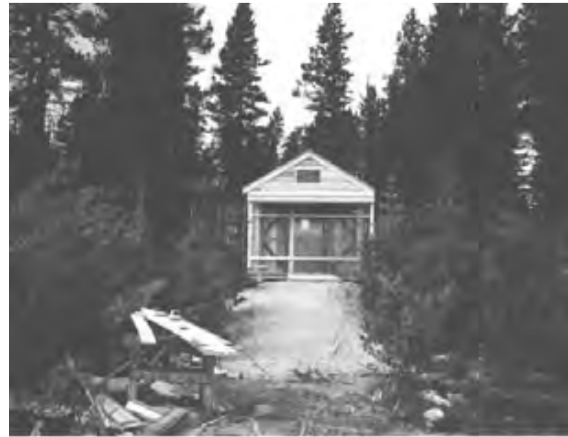
Figure 4: Log Cabin toilets
