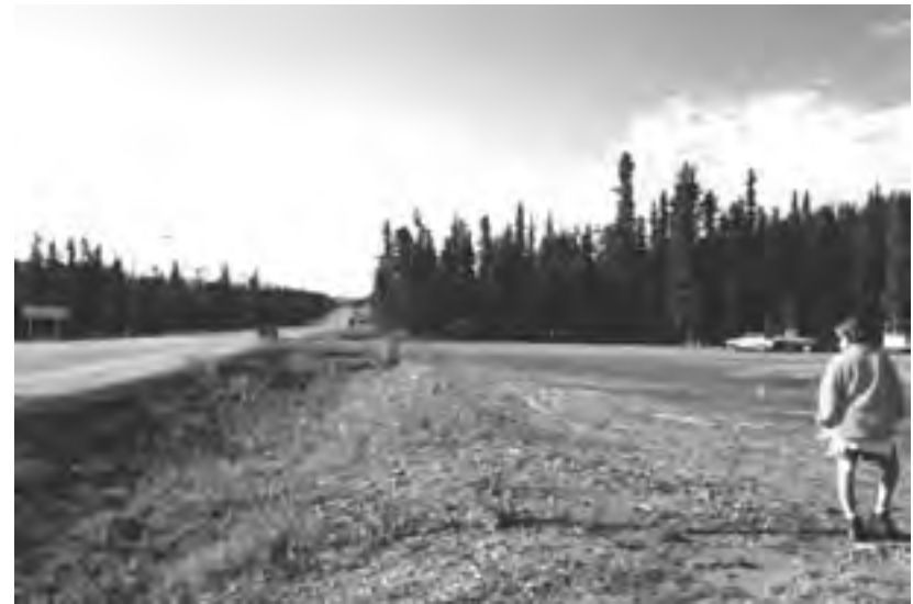
Figure 19: Carcross Road intersection facing east.
