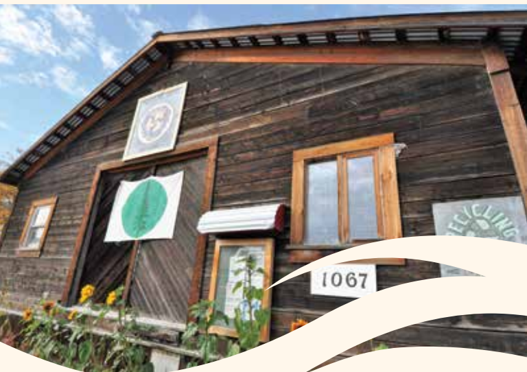
Strachan's warehouse YG photo
