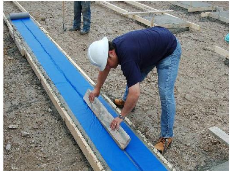
Figure 23. Capillary break using proprietary roll-applied material during casting of footing
