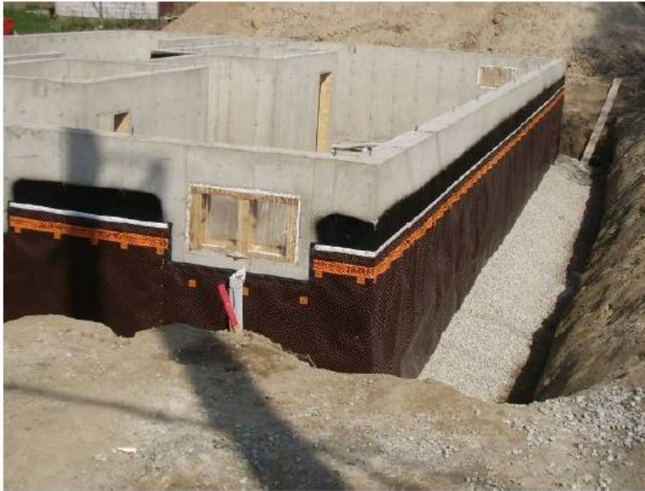
Figure 14. Air gap membrane applied over dampproofing on cast concrete wall
