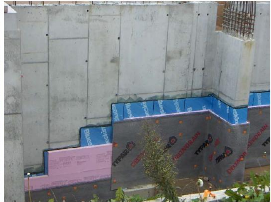
Figure 15. Air gap membrane applied over waterproofing membrane and insulation
