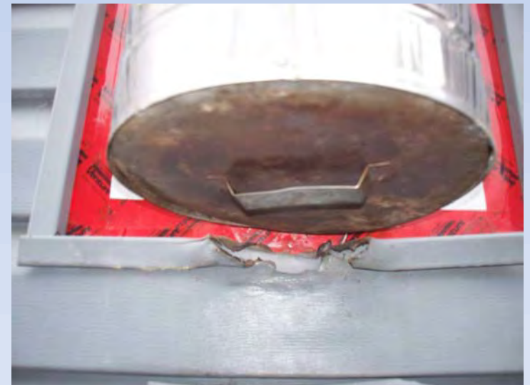
Less than required clearance
