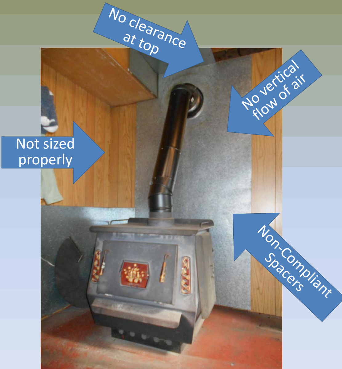
Non-compliant heat shields
