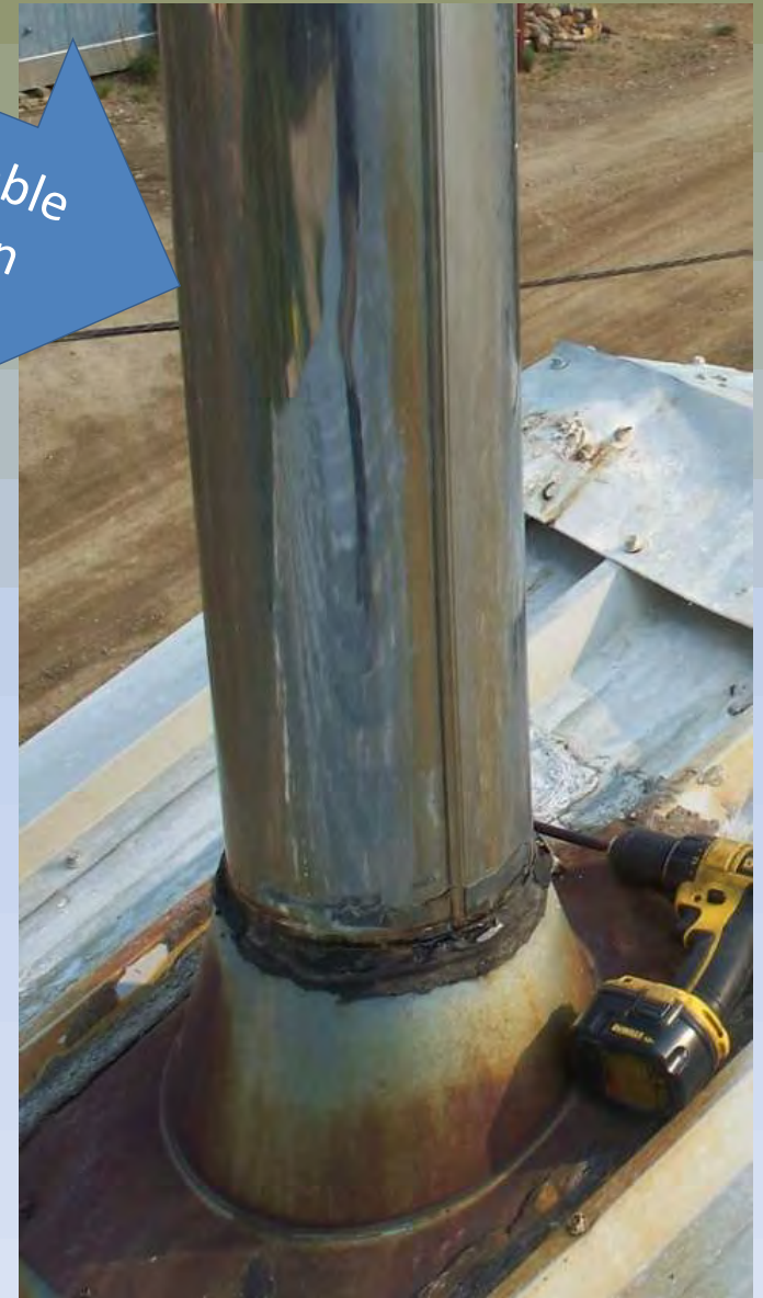
Outside view of chimney
