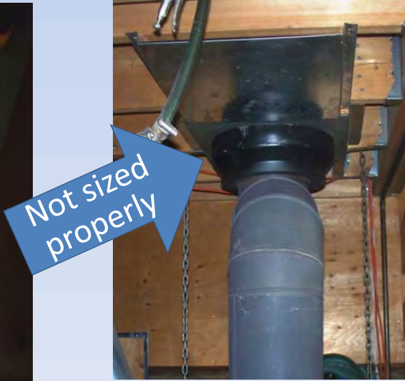
Non-compliant heat shields
