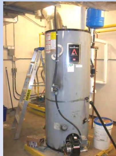
Oil-Fired Hot Water Tank
