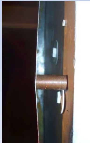
Non-compliant spacer
