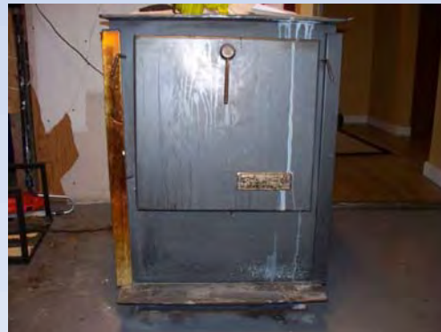
Firebox highly deteriorated
