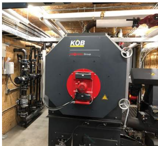
Figure 2-10 - Yukon Garden's Biomass Boiler
