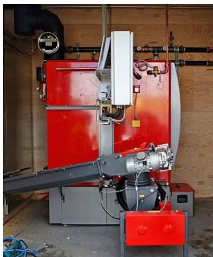
Figure 2-7 - Teslin Biomass Boiler
