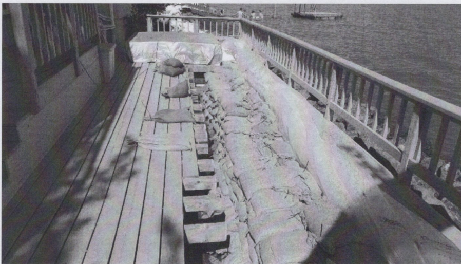
Photo 3. Typical Sandbag dike
