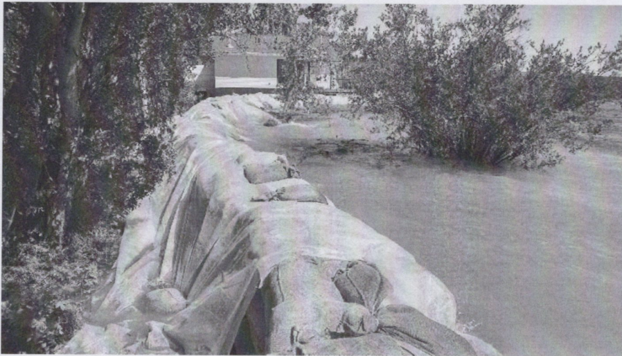
Photo 4. Typical Sandbag Dike
