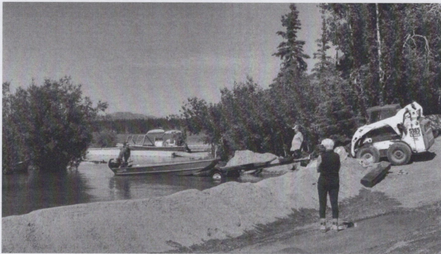
Photo 1. Early Earth Dike of Sand and Gravel.
