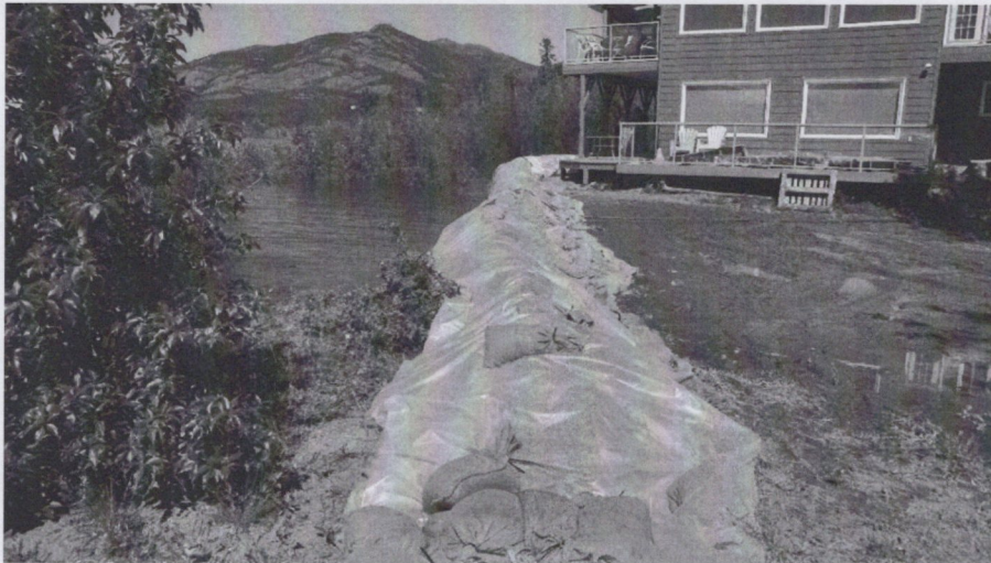
Photo 2. Typical Sand and Gravel Dike, Wrapped in Poly.
