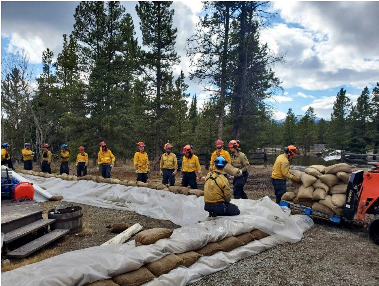
Photo 5: Wildland Fire Management (WFM) responders construct a berm at Gem Haven to protect local residents and agricultural land. Historically overland flooding at Gem Haven has not been an issue and was an early indication of possible flooding to come.
