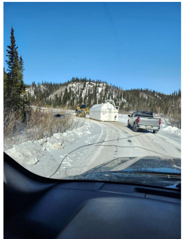
Photo 4: Moving old fuel tanks from the fuel tank farm to prevent damage to critical infrastructure in the event the empty tanks are moved by flood waters.
