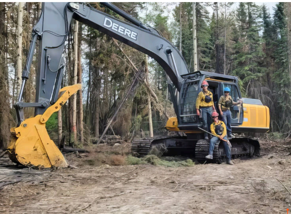
Berdoe crew (Joey Powell, Jesse Globensky and Parker Almond) poses on an excavator while on export in Alberta. Photo by Joey Powell
