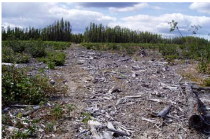
Summer road construction
