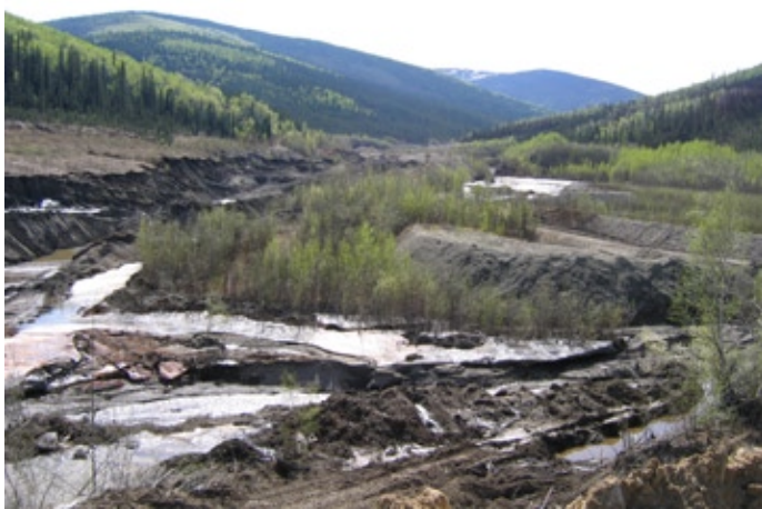
Results of stripping and trenching activities in an operating placer mine. (Photos courtesy of Mineral Resources Branch)
