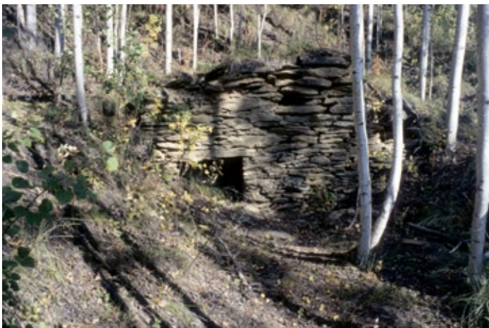
Foundation with stone fireplace. Eldorado Creek
