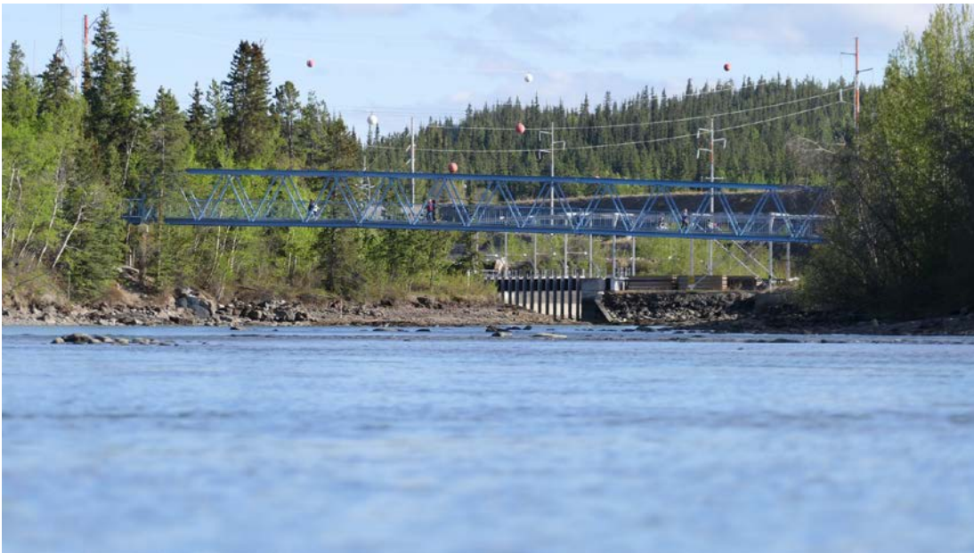
Downstream view of the Whitehorse Rapids hydroelectric facility and Rotary Centennial Bridge
