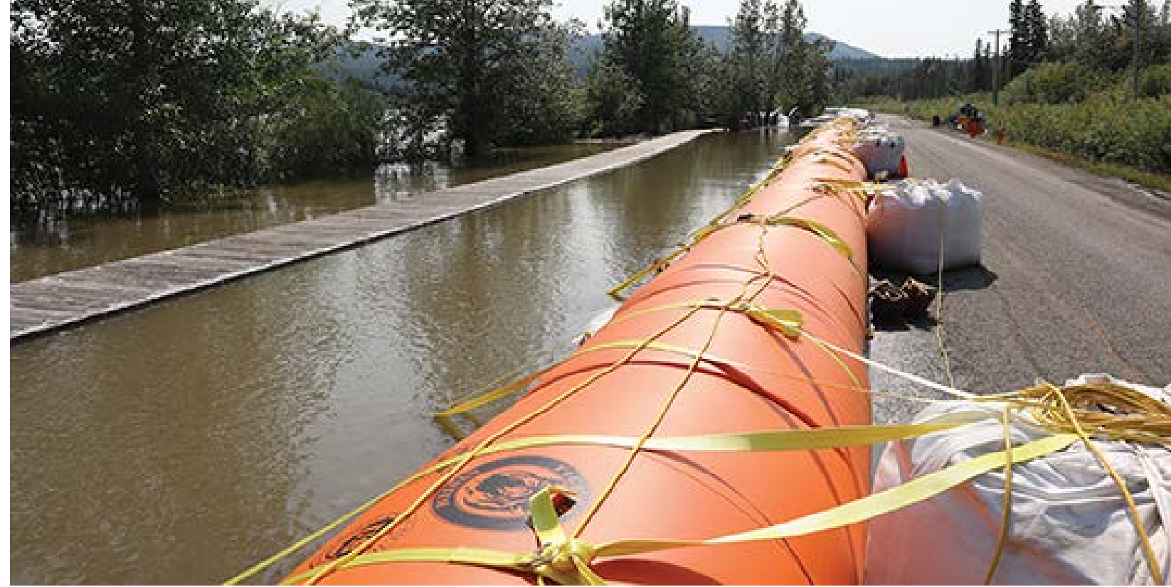
A Tiger Dam 3 set up on River Drive in Carmacks, Yukon (Anthony Bier, 2022)
