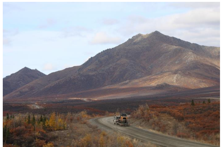
Construction equipment on the move.
