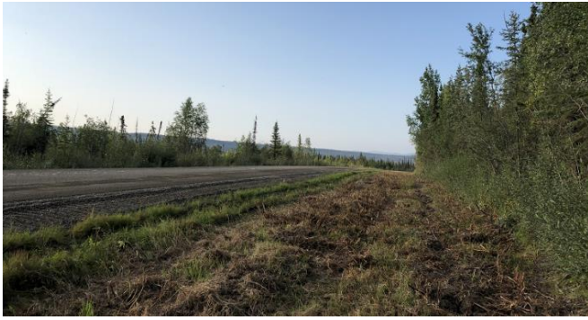
Completed section of the conduit installation
