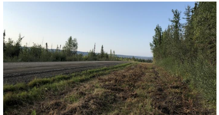
Completed section of the conduit installation
