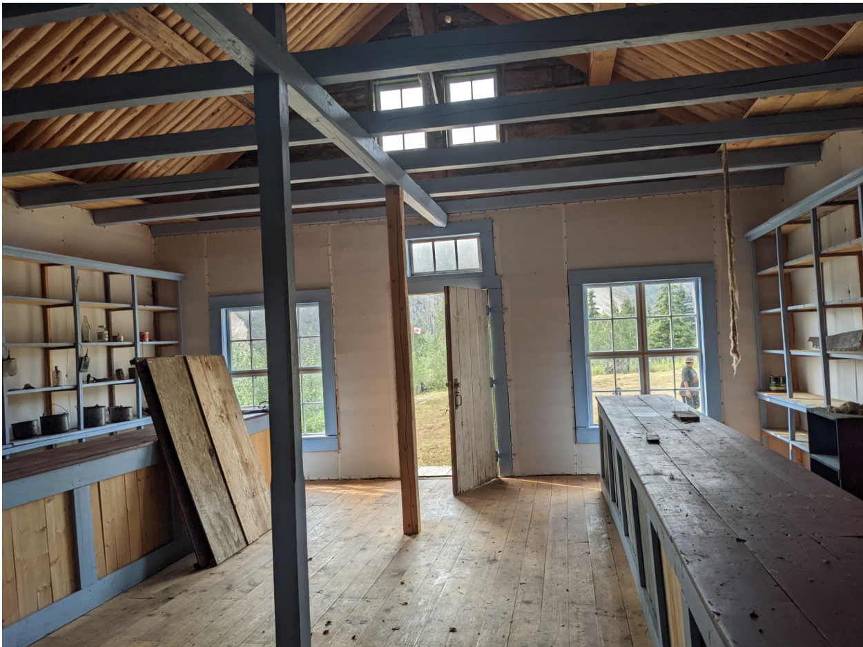
Interior of Cadzow's Store, Rampart House, 2022. Wendy Shearer photo
