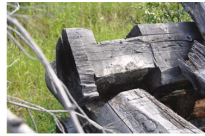
Notch detail of collapsed cabin at LaPierre House, n.d. YG photo
