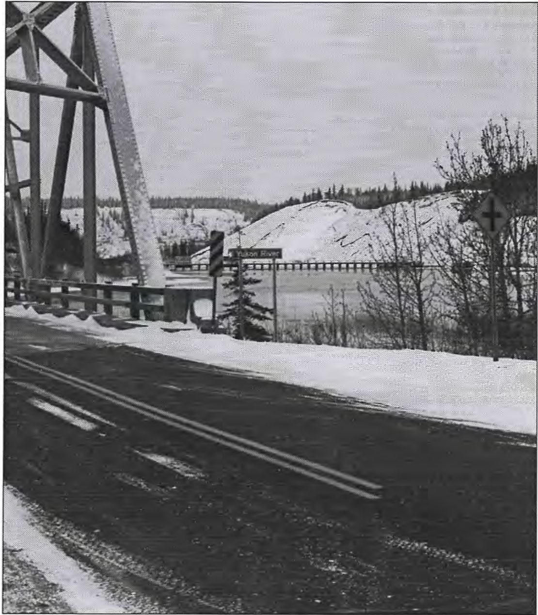
Yukon River bridge site with a view of the marsh lake dam.
