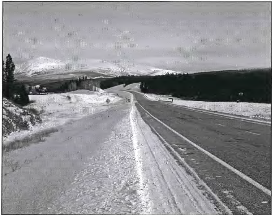
Swift River Crossing, km 1168.
