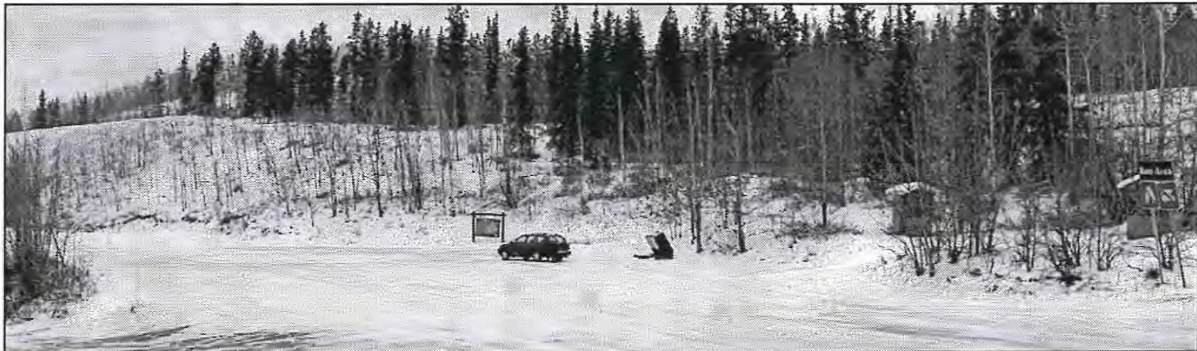
Marsh Lake Dam rest area at south end of bridge, km 1443.
