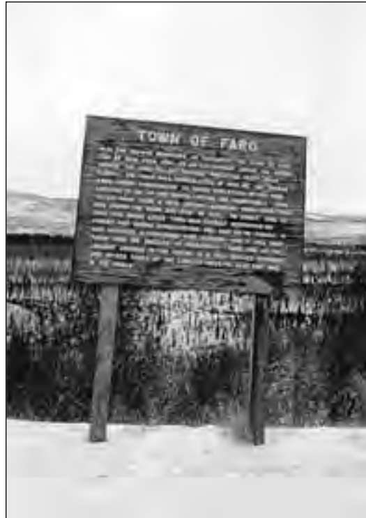
Above, the older Canol Road sign has weathered better than the Town of Faro sign. The latter displays serious problems with its varathane finish.
