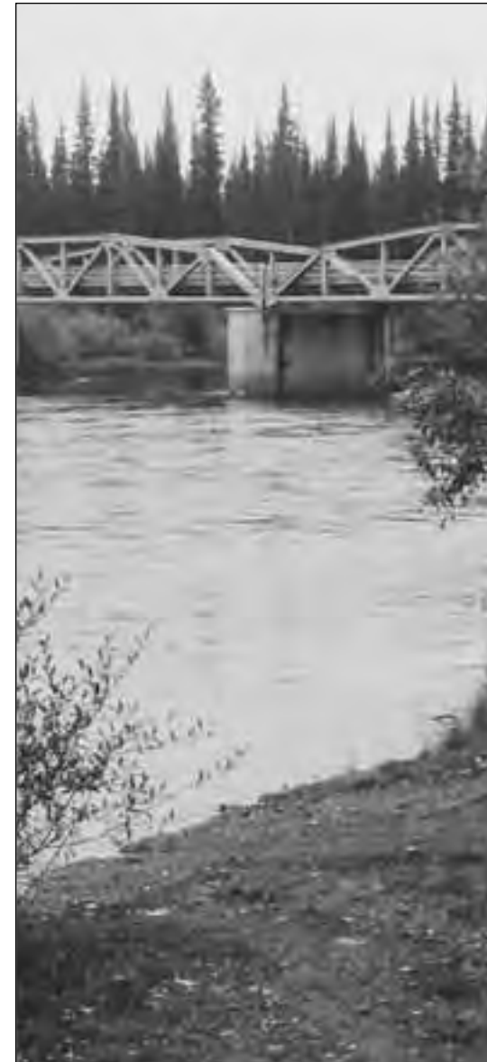
View of Francis River Bridge from the boat launch.
