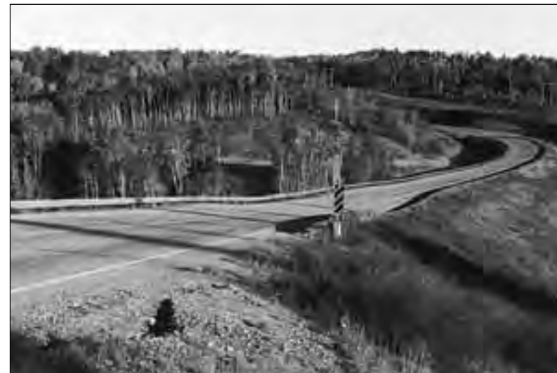
An upgraded section of the Campbell Highway, North of Faro.
