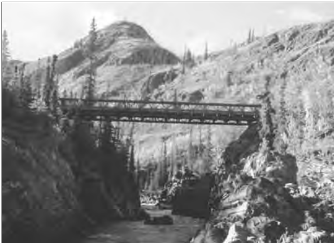
The Lapie River Bridge.
