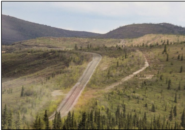
Photo 6 - ToW Highway and remnants of the 1930-40's road (Photo: NVision)
