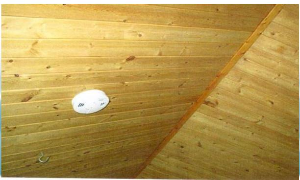
When a a fuel-fired appliance is installed or replaced in a building with a residential or care occupancy, the National Building Code (NBC) also requires that smoke alarms and carbon monoxide (CO) alarms be installed in conformance with the NBC.
