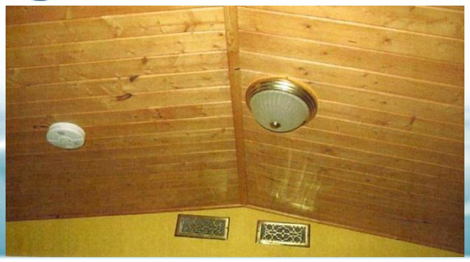
When a a fuel-fired appliance is installed or replaced in a building with a residential or care occupancy, the National Building Code (NBC) also requires that smoke alarms and carbon monoxide (CO) alarms be installed in conformance with the NBC.
