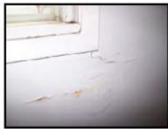
Water-Damaged Drywall
