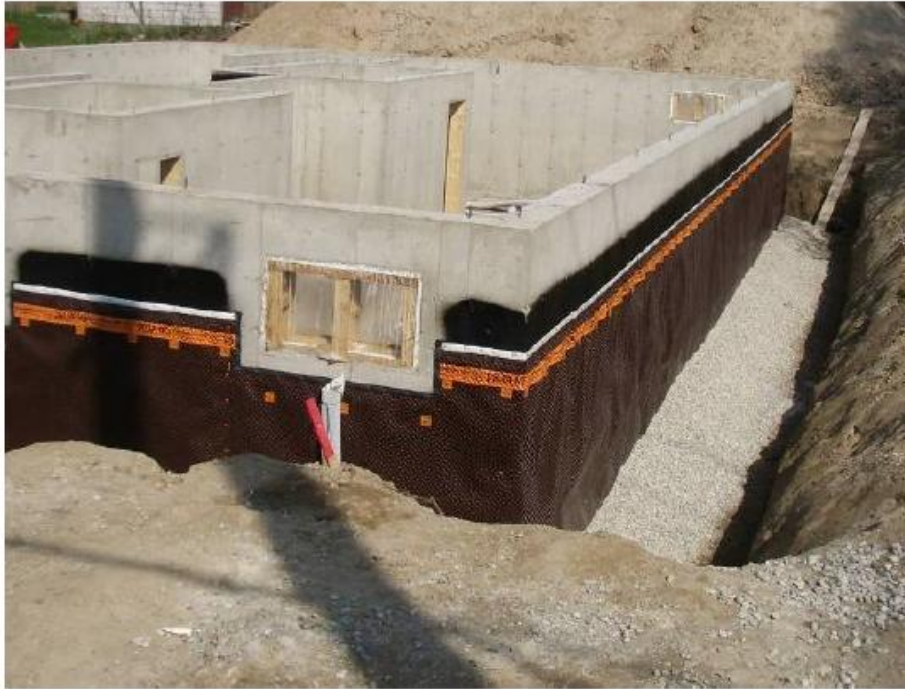
Figure 14. Air gap membrane applied over damproofing on cast concrete wall
