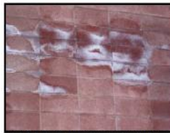
Mineral Deposits (Efflorescence) on Tile
